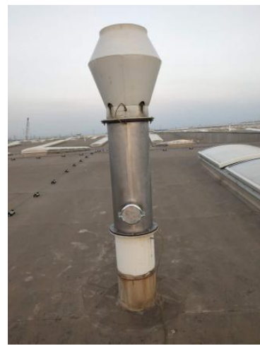
抛丸废气排气筒P62
