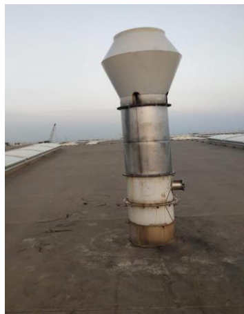
抛丸废气排气筒P63
